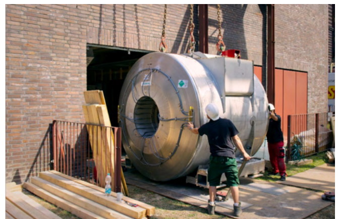
Fig. 1: Delivery of the new 7T MR system in August 2020. The new magnet is considerable shorter than the previous magnet but, due to active magnet shielding, is slightly larger in diameter. Just small enough to enter the ELH.
