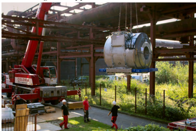
Fig. 1: Delivery of the new 7T MR system in August 2020. The new magnet is considerable shorter than the previous magnet but, due to active magnet shielding, is slightly larger in diameter. Just small enough to enter the ELH.
